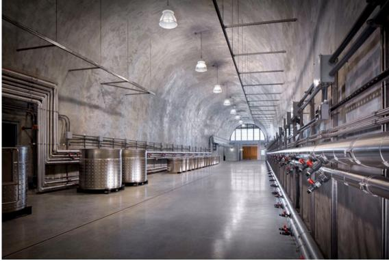
The winemaking regimen is very traditional with rigorous sorting, whole cluster fermentations, native fermentations, and foot crushing. Temperature-controlled fermentation tanks are supported by utility stations and are uniquely designed to allow pressing in the fermentation tank. There are no pumps in the winery and the wines are never filtered. Wines are barrel aged for 18 months in 70% new three-year air-dried Francois Frères barrels and aged in bottle for at least two years.
